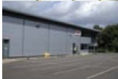
Building prior to demolition
